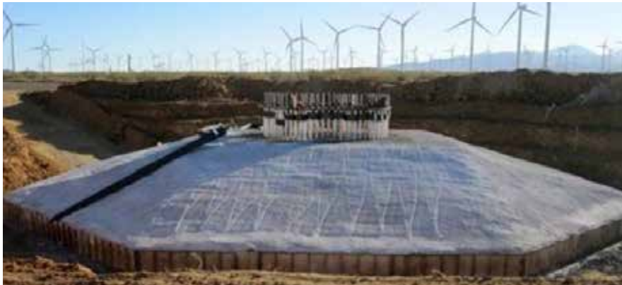
Wind Turbine Foundation Design
